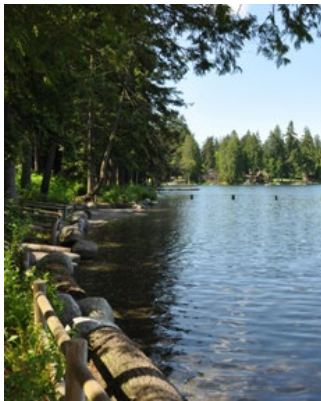
Logs and boulders protect the shoreline along Pine Lake (credit: Eric Willhite)
