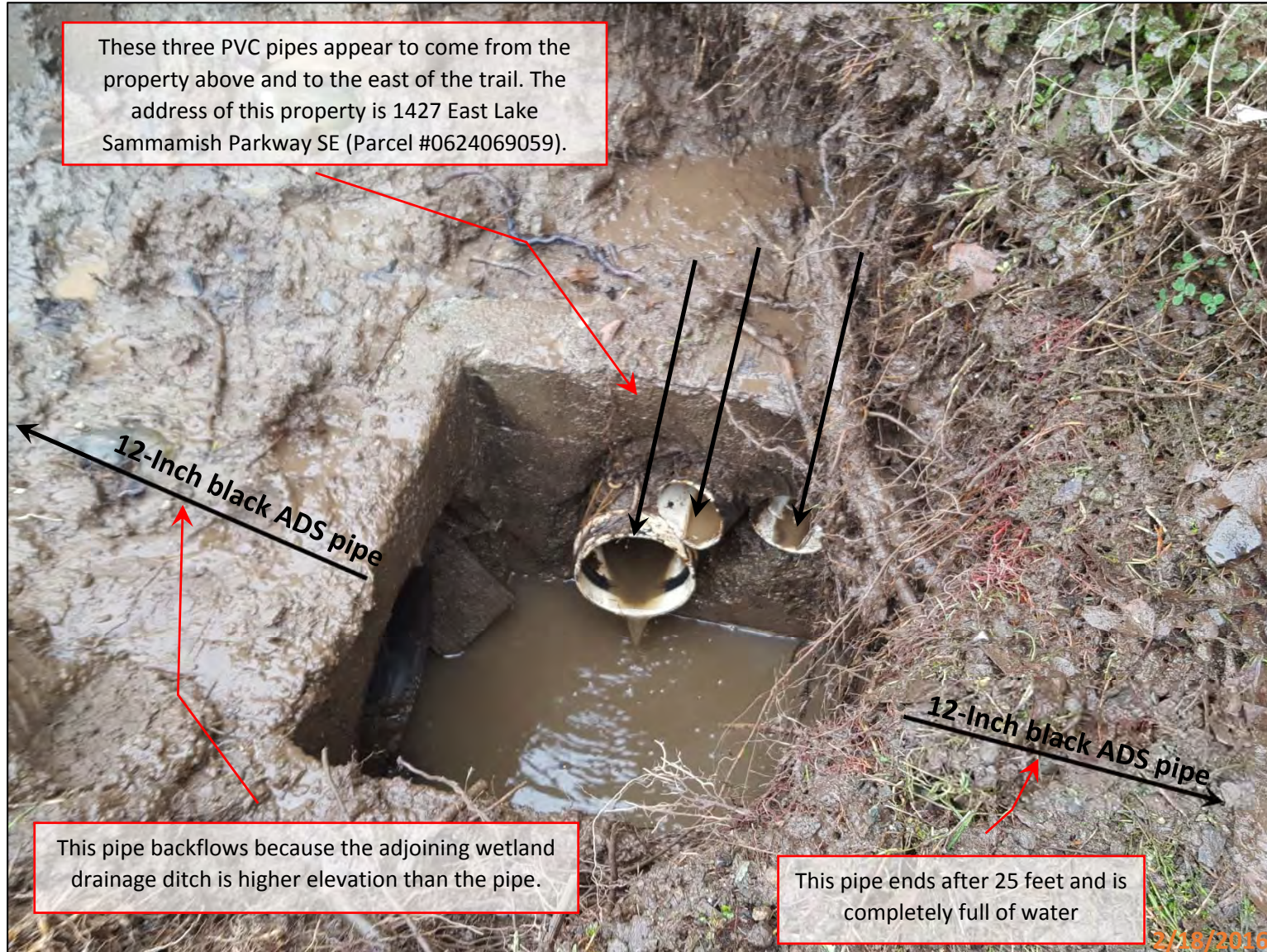
Picture 4 - This picture shows the drainage structure from Picture 3 after it was cleaned out with a vector truck. The large white pipe on the left is a 6-inch PVC pipe and the other two white pipes are 4-inch PVC pipes. There are also two 12-inch diameter black corrugated ADS pipes that connect to this structure. This structure does not have a lid. None of the pipes observed in this structure appear to have been tightly grouted at the opening in which they enter the concrete structure. This is common construction practice.
