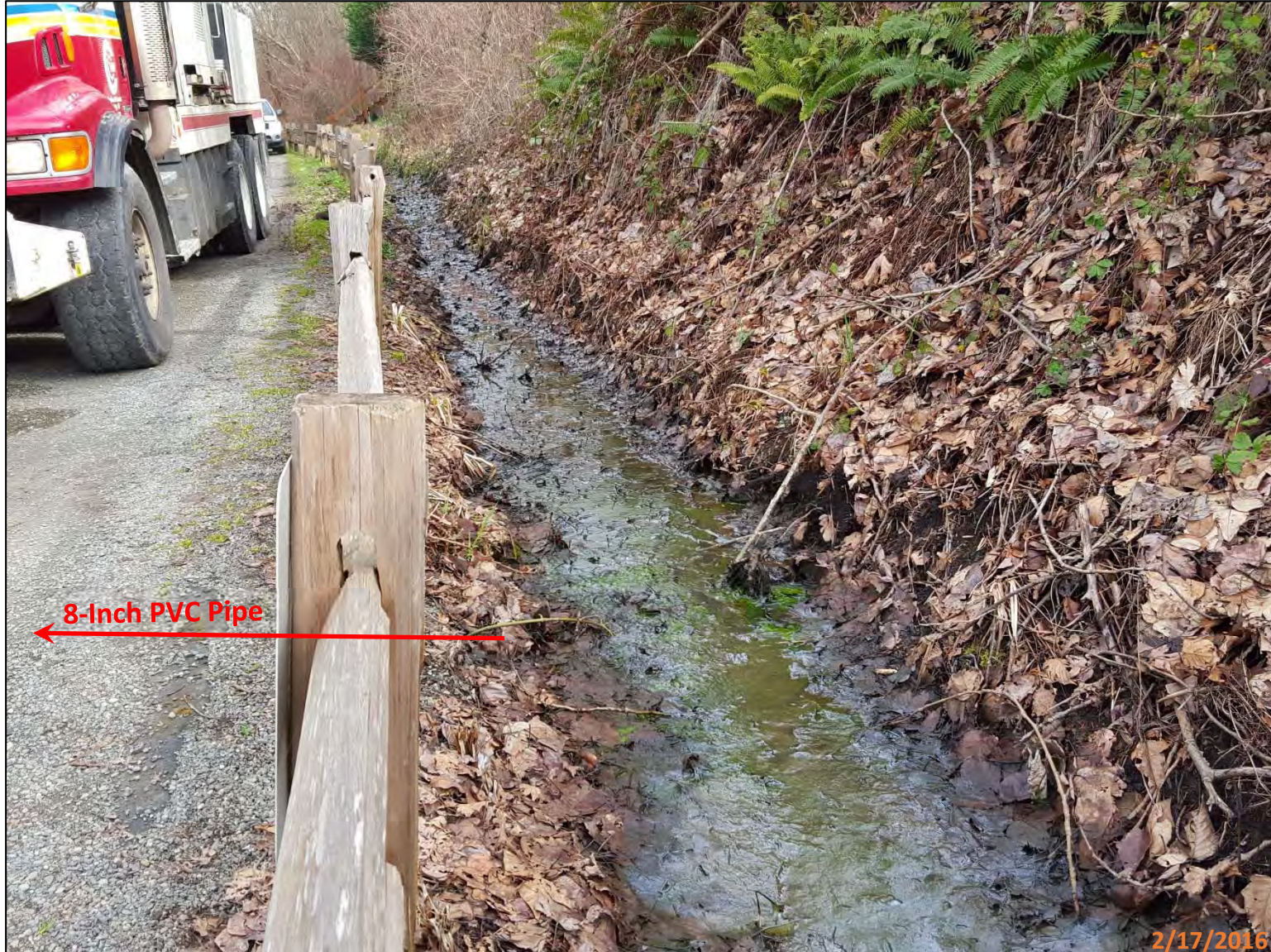
Picture 6 – This picture shows the drainage ditch/wetland approximately 20-to-30 feet north of the drainage system shown in pictures 1-5. This ditch water backflows into the drainage system because the ADS pipe shown in Picture 1 and 2 is lower in elevation than the drainage ditch. There is also an 8-inch PVC pipe that travels beneath the trail and connects to a yard drain in front of 1428 E Lake Samm Shore Ln SE (shown in red). See Picture 7-10 for more information on this drainage pipe. (Looking north)
