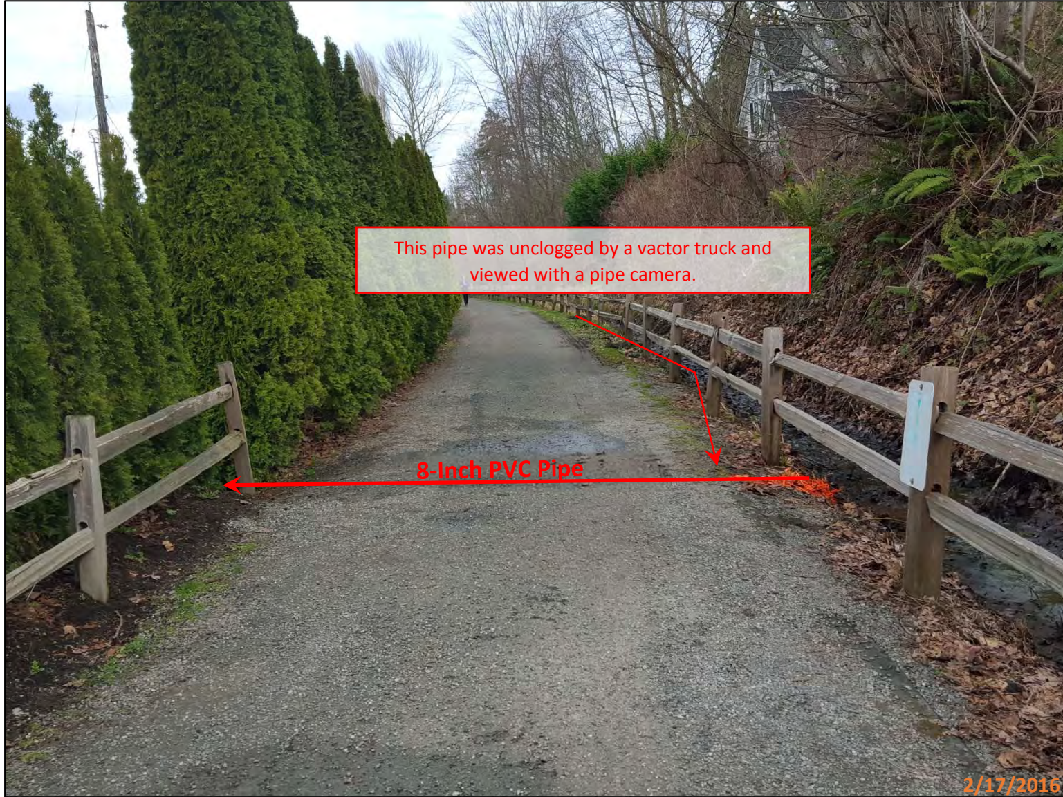
Picture 7 – This 8-inch PVC pipe travels west from the drainage ditch and enters a yard drain in front of 1428 E Lake Sammamish Ln SE. (Looking north)
