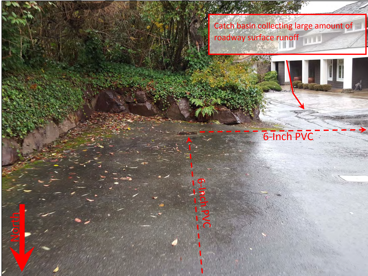
Picture 3 – This picture shows another catch basin on East Lake Sammamish Shore Ln NE. (Looking south from East Lake Sammamish Shore Ln NE)
