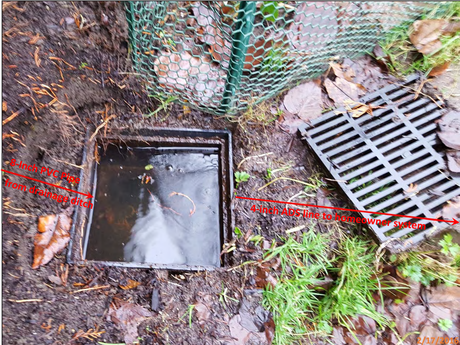
Picture 9 - This picture shows the yard drain prior to the vacor truck cleaning it out. This is the location that appears to overflow in heavy rain events. Onto East Lake Sammamish Shore Lane SE. This area received a complaint from the Tsilas Residence on 1/19/2016. The water in the yard drain appears to be at least 12-inches above the crown of the 4-inch ADS outlet pipe. The pipe does not appear to be draining. The orientation of the 4-inch ADS line is unknown.
