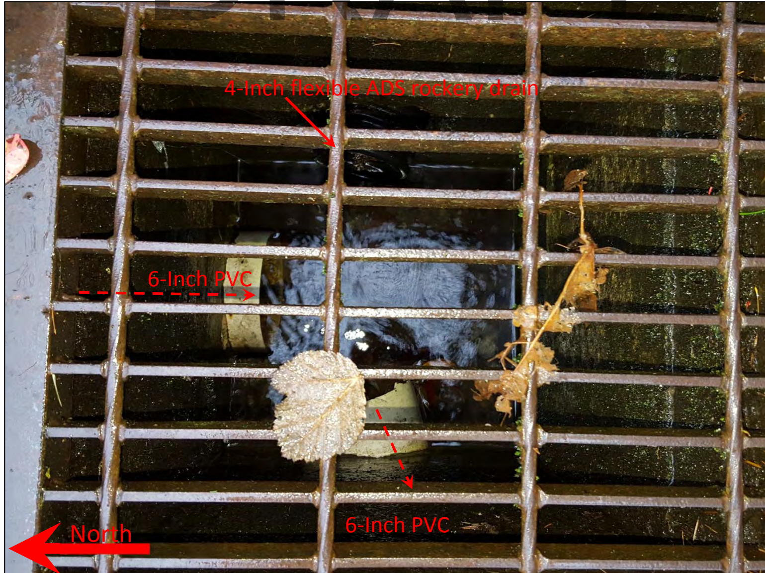
Picture 4 – Looking downward at the catch basin from Picture 3 on East Lake Sammamish Shore Ln NE. The water continues through the 6-inch PVC pipe. The black pipe on the top of the picture is a 4-inch ADS pipe that appears to come from the rockery to the east. (Looking downward and facing east from East Lake Sammamish Shore Ln)
