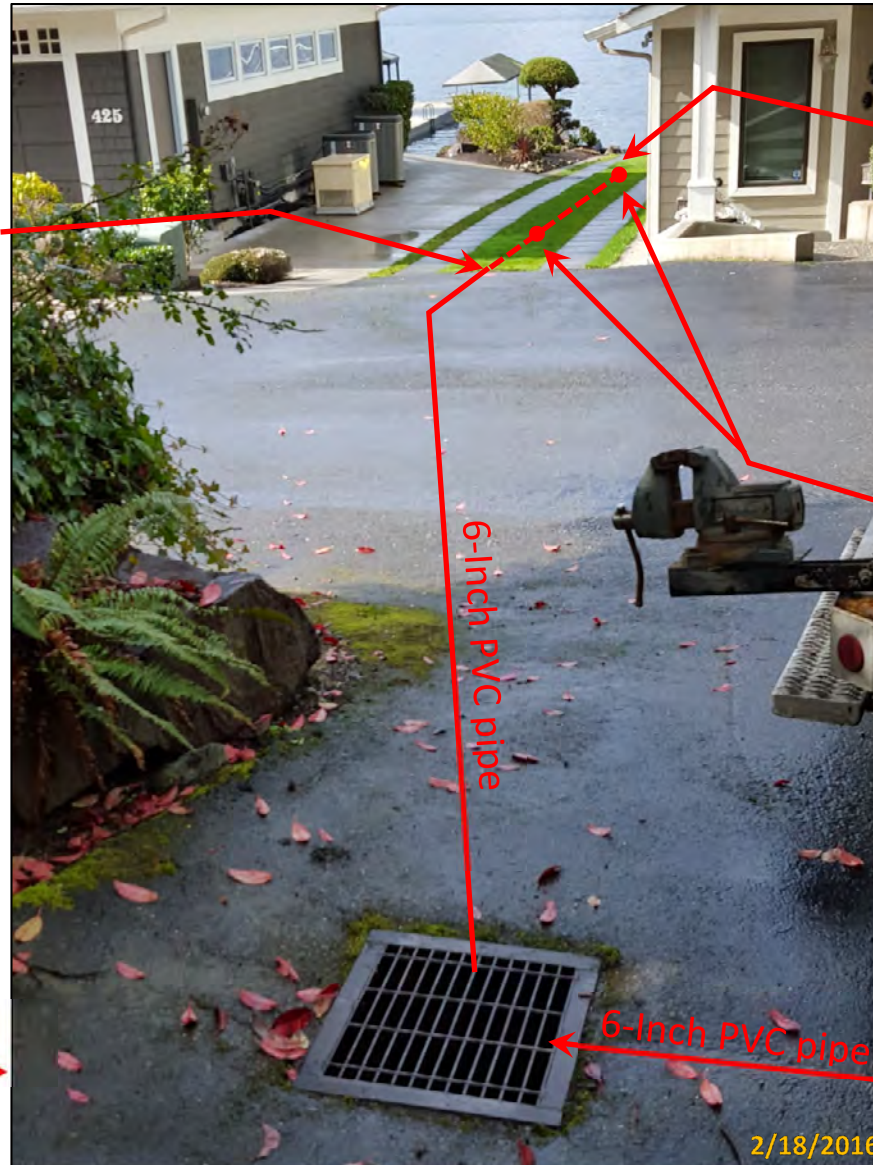
Picture 1 – This picture shows the 6-inch PVC pipe that was TVed with a camera. The 6-inch PVC pipe shown in this picture is a solid wall white PVC pipe until the pipe reaches the homeowner’s grass. At the grass, the pipe transitions to a 6-inch perforated PVC drain pipe. (Looking west from East Lake Sammamish Shore Ln NE)
