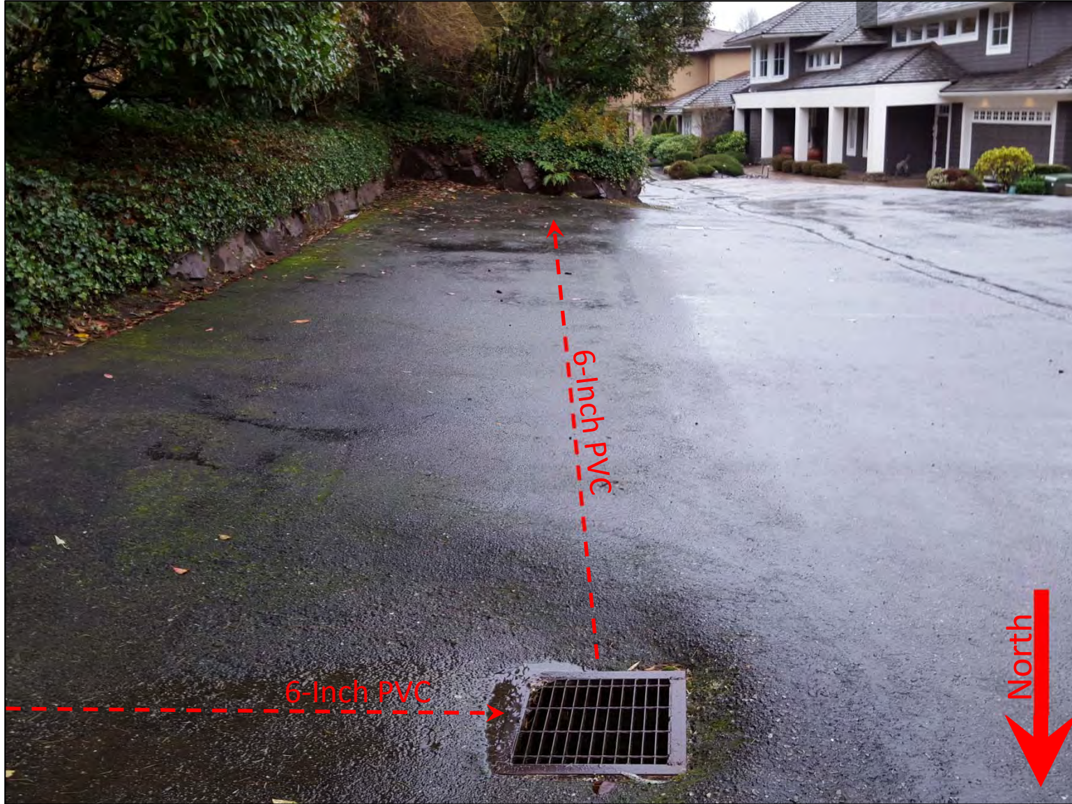
Picture 2 – This picture shows another catch basin on East Lake Sammamish Shore Ln NE. On the right side of the picture you can see a large amount of run-off from the East Lake Sammamish Shore Ln NE. This is the same catch basin shown in picture 1. (Looking south from East Lake Sammamish Shore Ln NE)
