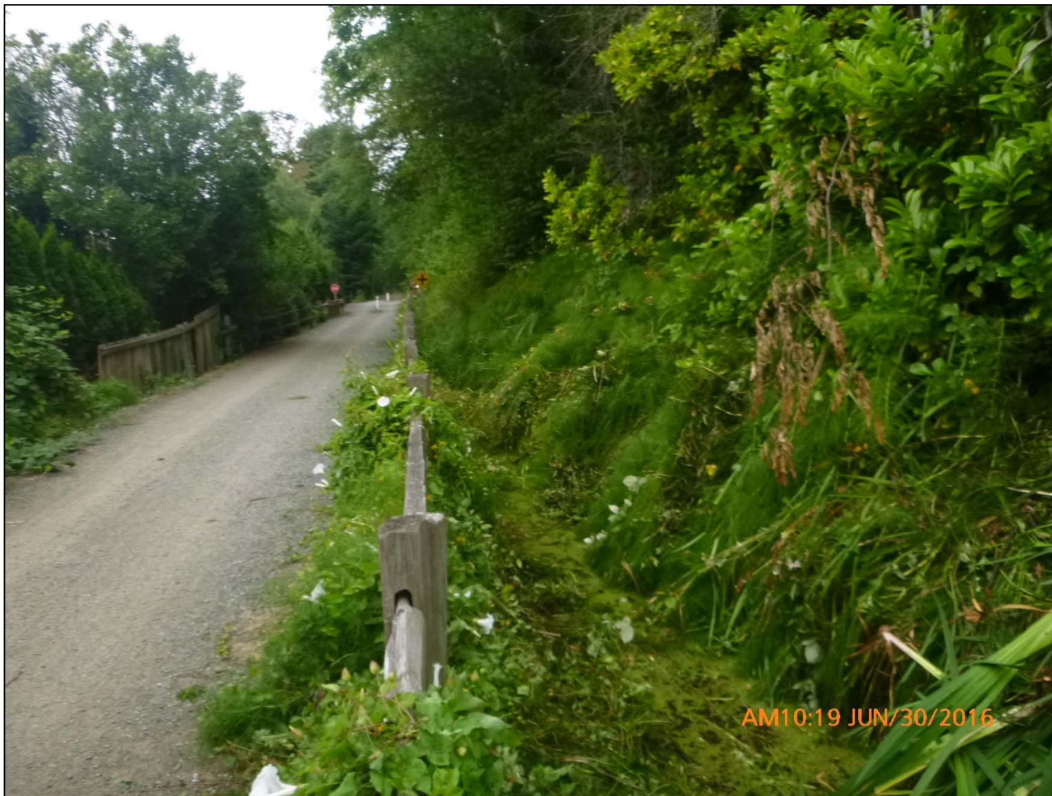
Picture 2 - This photo shows the ponding water in the wetland directly in front of Mr. Hill's property. This wetland is on the east side of the trail and cannot drain due to the clogged pipe shown in picture 1. (Looking south)
