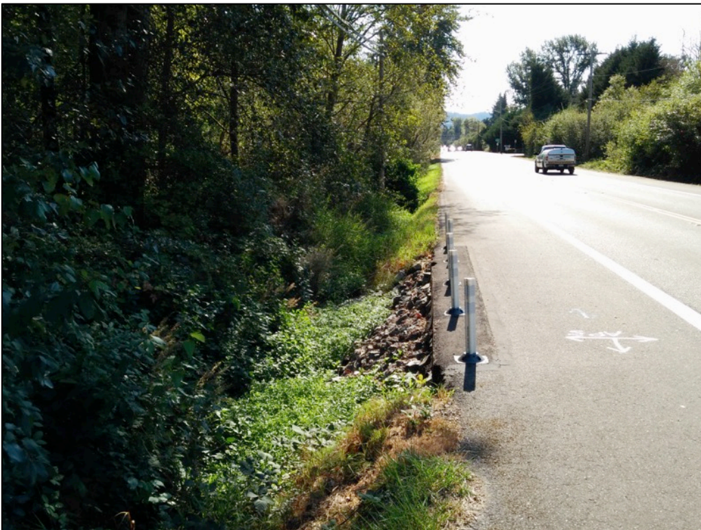
Figure 18. View of the Zackuse Creek culvert on the eastern margin of East Lake Sammamish Parkway; view is to the south.
