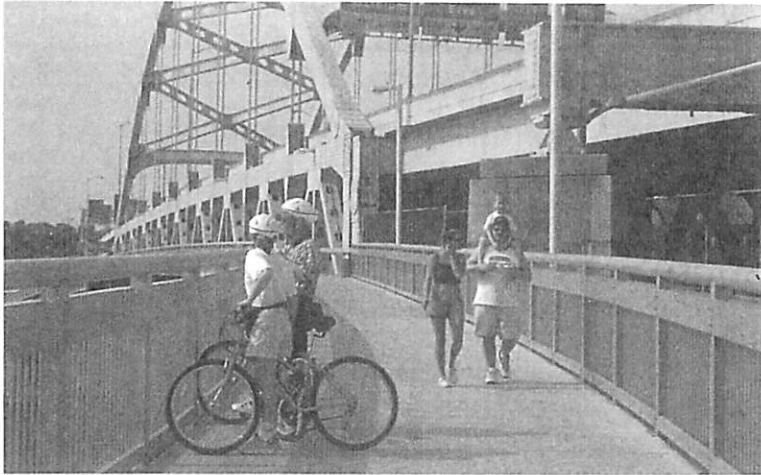
Figure 5-12. Example of Bridge Structures (Photo courtesy of Jennifer Toole of Toole Design Group.)
