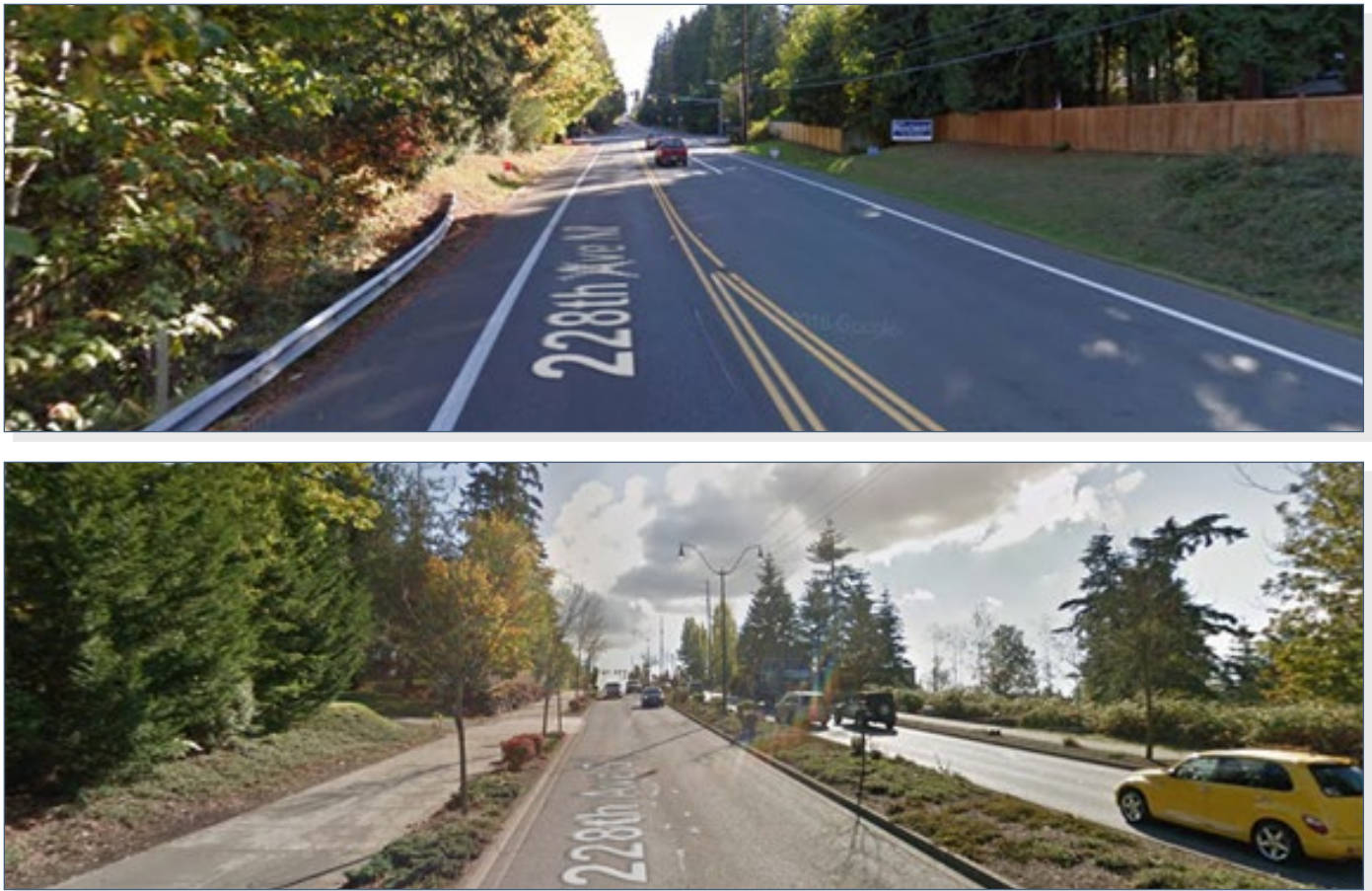
Figure 10. Unimproved Section (top) and improved Section (bottom) of 228th Avenue SE. Source: Google Maps.
