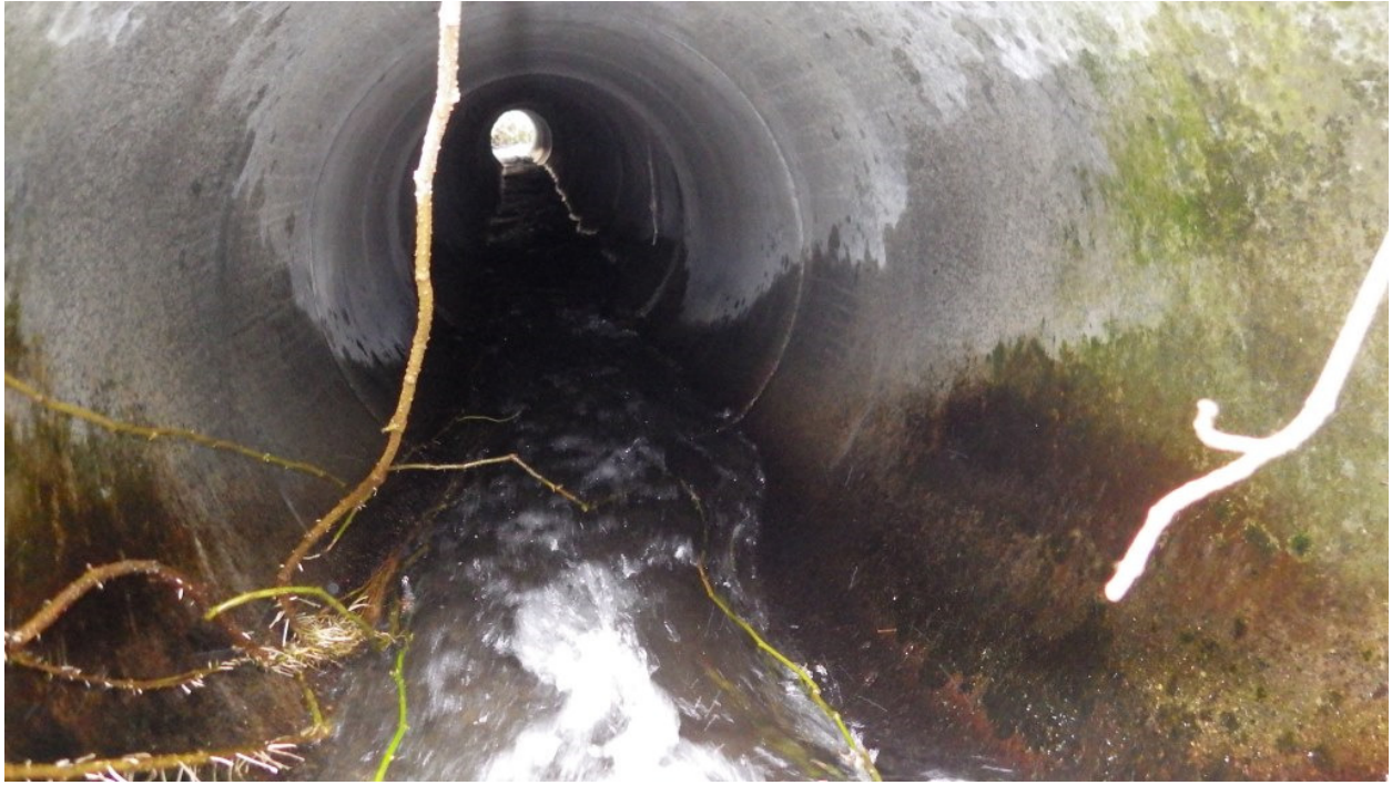
culvert lacks substrate
