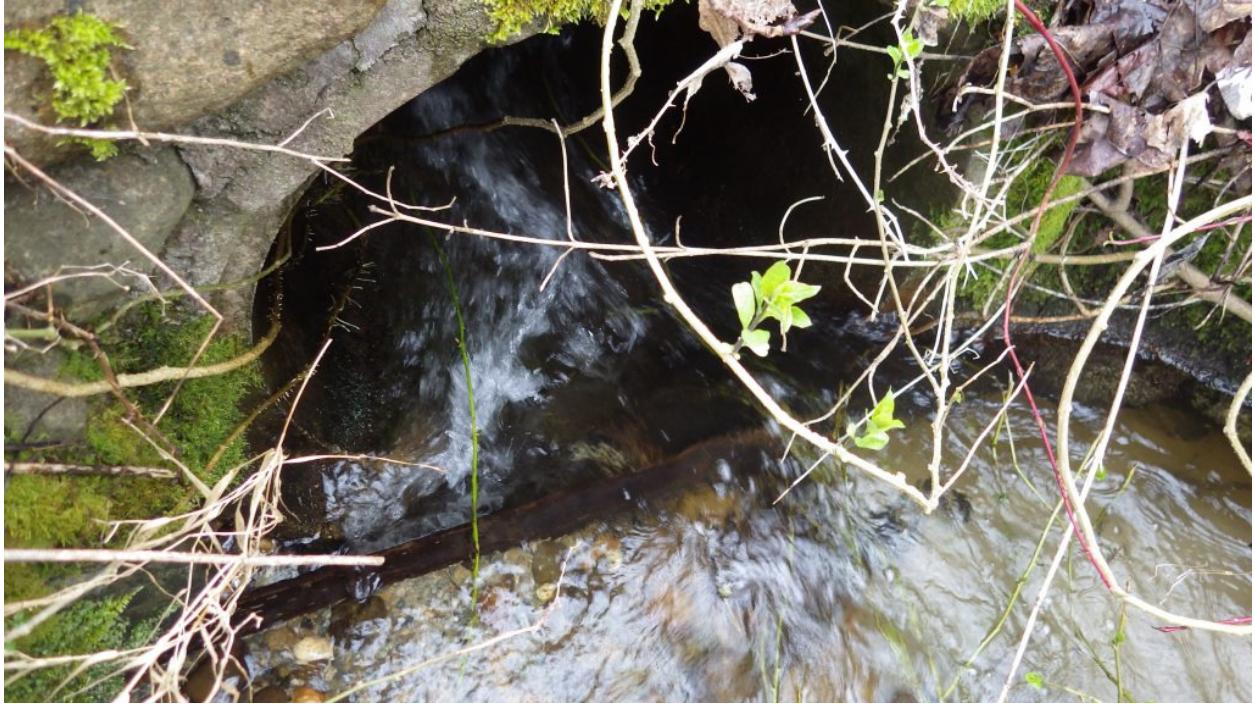
culvert lacks substrate
