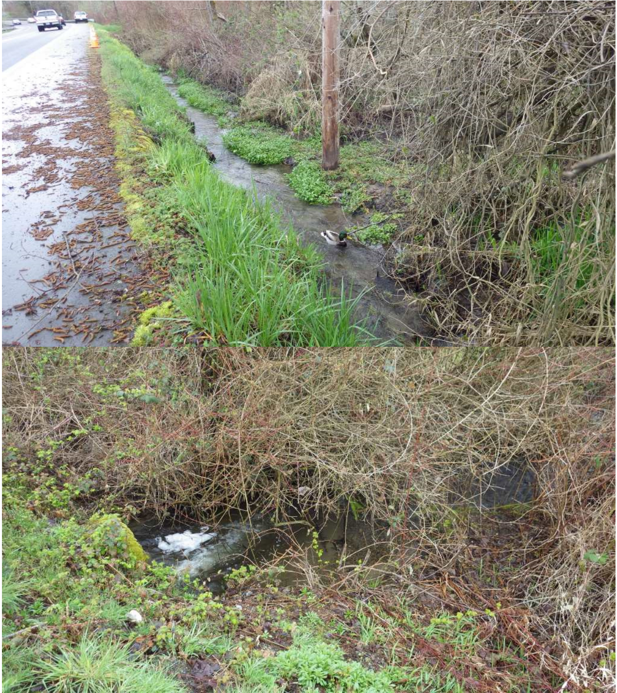
culvert downstream of ELSP
