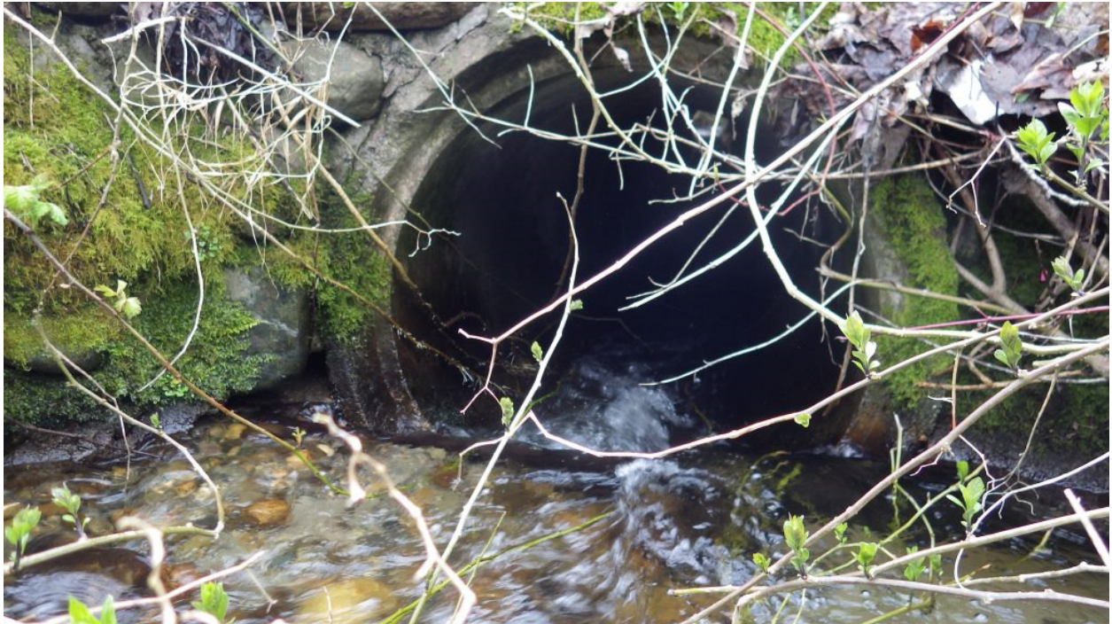
culvert inlet (30 inch concrete) under ELSP; identified as a partial barrier by WDFW; site ID 920253
