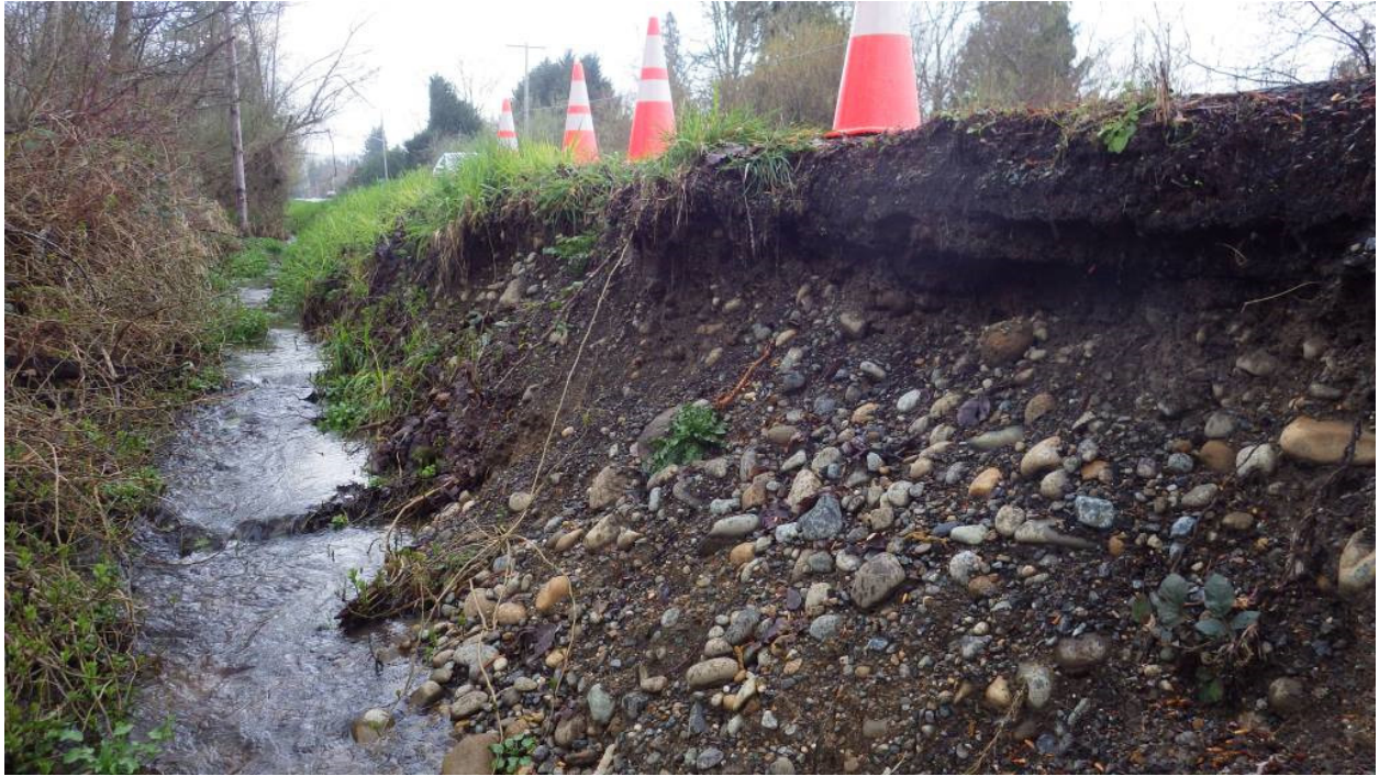
channel was approx. 6 ft wide with 5 feet wetted (BFW 7 ft downstream), approx. 3% slope
