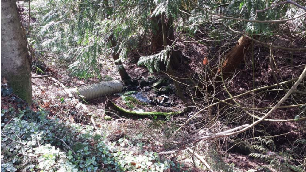
Zackuse Creek Outfalls
