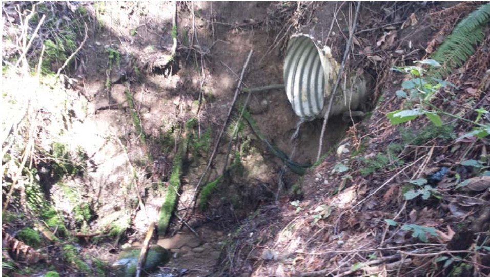
Zackuse Creek Outfalls
