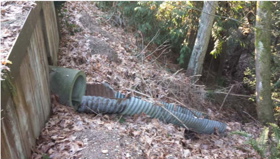
Zackuse Creek Outfalls
