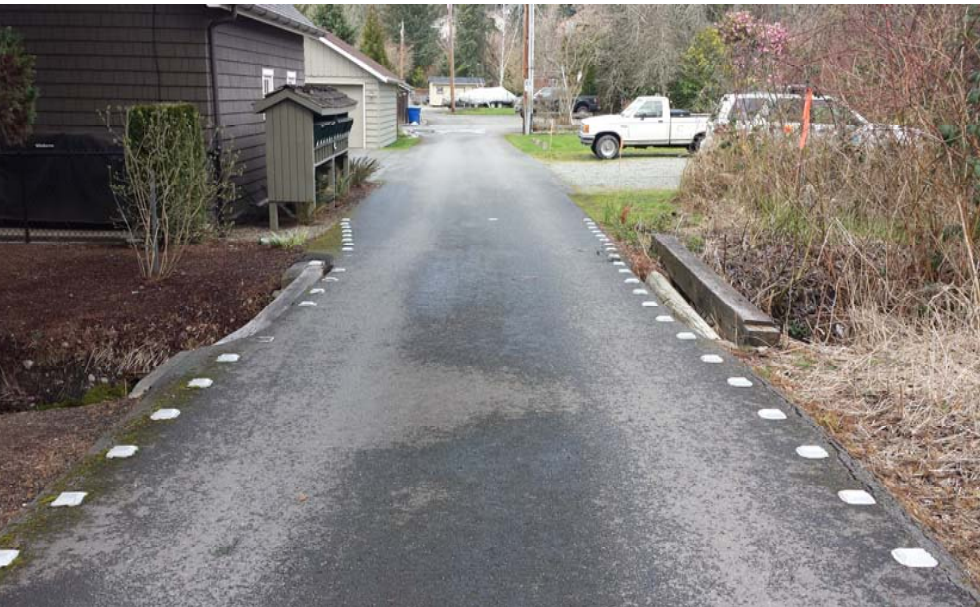
Culvert at East Lake Sammamish Shore Lane
