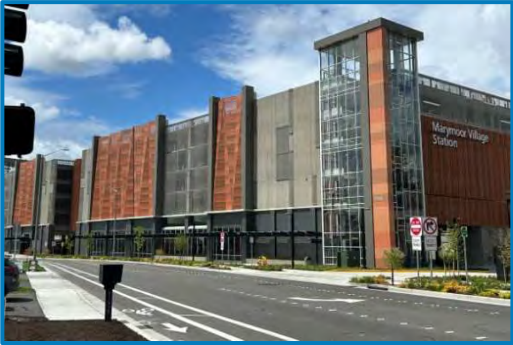
FIGURE 36. BUFFERED BIKE LANE IN REDMOND, WA
