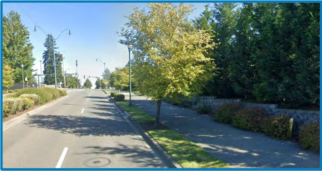
FIGURE 38. SHARED USE PATH ALONG 228 TH AVENUE SE, SAMMAMISH, WA
