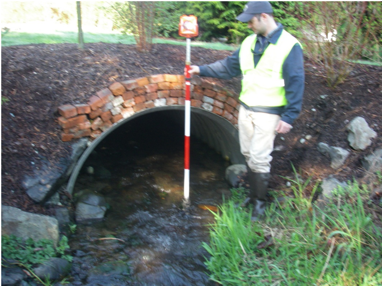
Figure 1. Surveying Zaccuse Creek Center Line at the Upstream End of the 5'-6" Corrugated Metal Pipe (CMP) Culvert, at the Downstream End of the Survey (Station 0+00).
