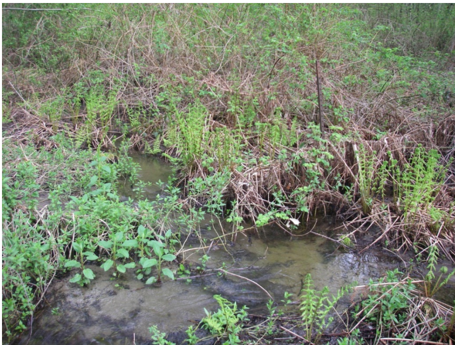
Figure 9. Multiple Channels in Low Gradient Depositional Area Influenced by the Culverts.
