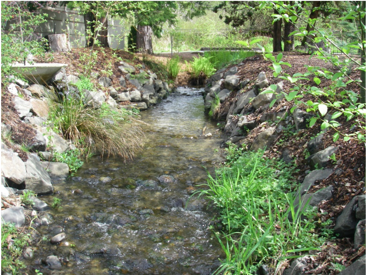
Figure 2. Looking Upstream Through Reach 1 with Riprap Banks on Both Sides.
