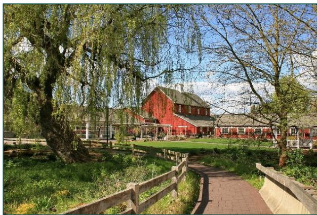
Exhibit 16: Pickering Barn Exterior
