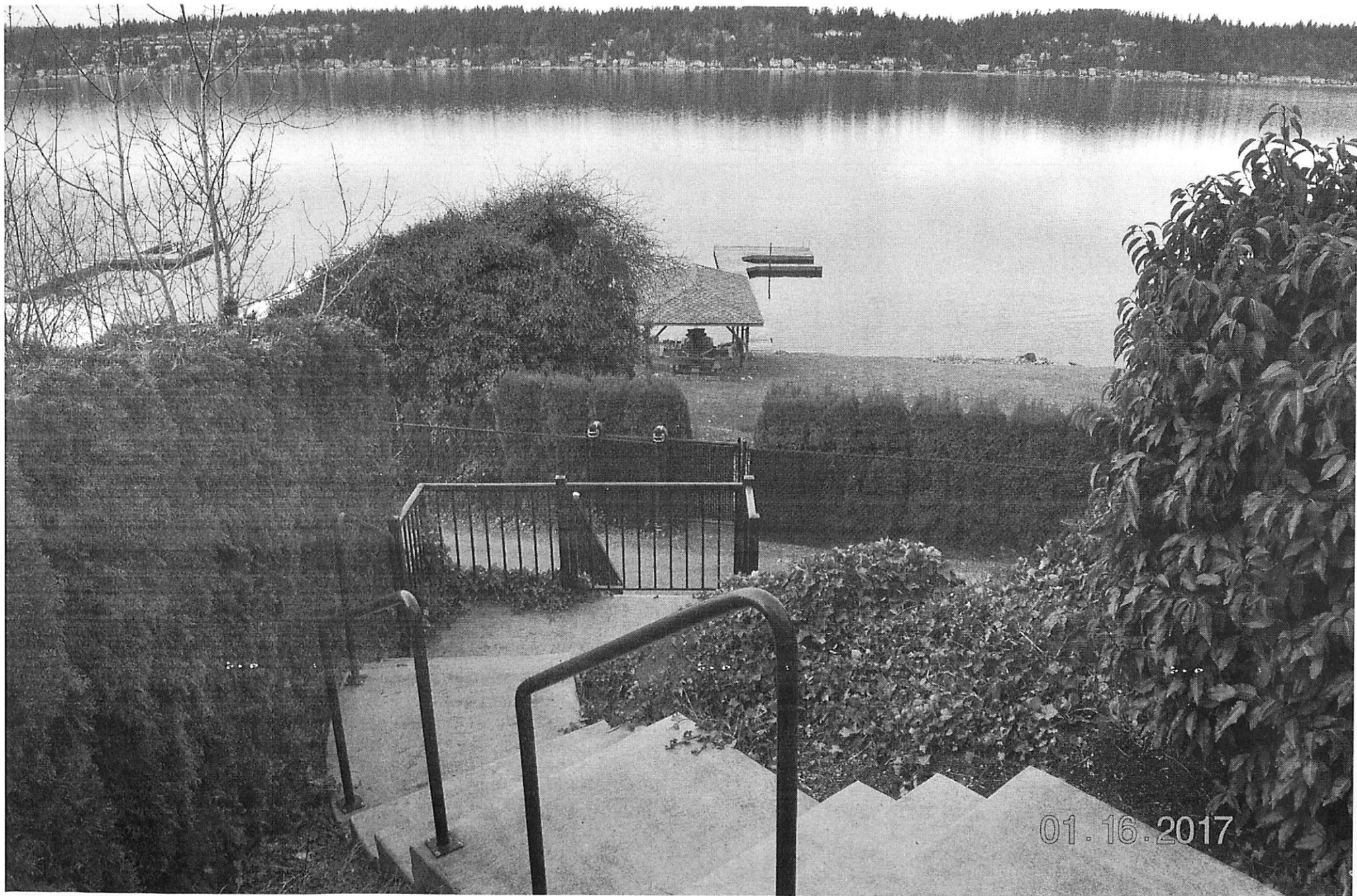
Concrete Steps Down To Wooden Steps
