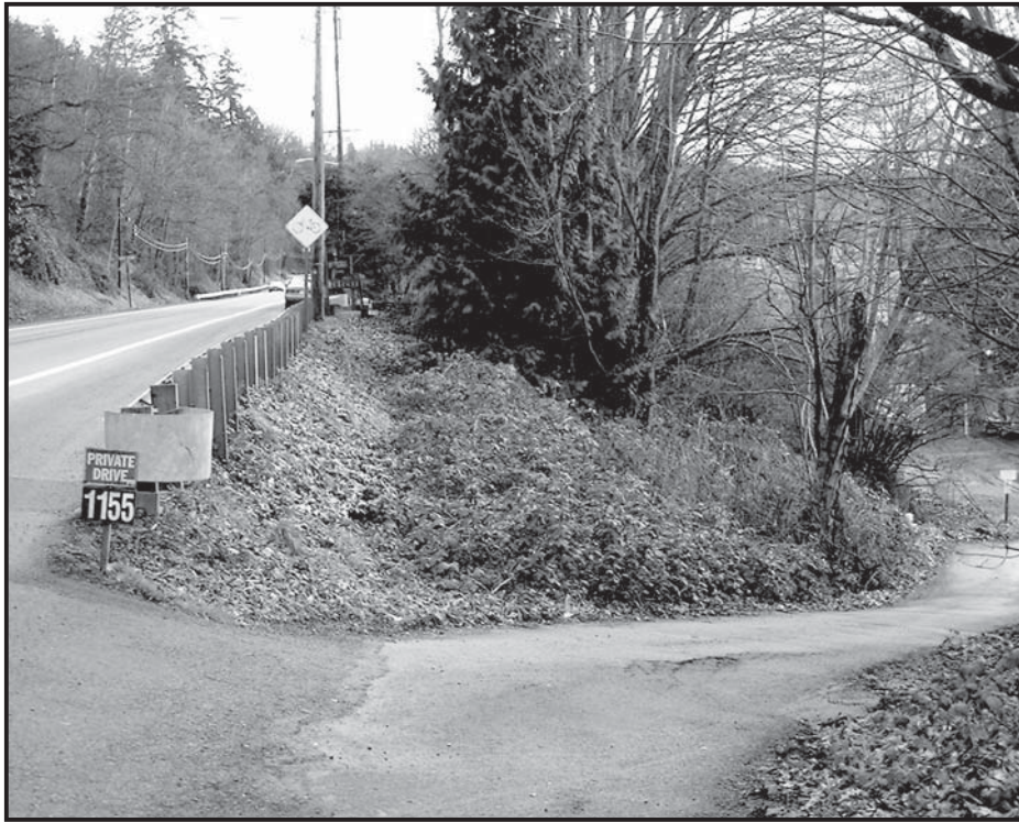
Looking south from first driveway south of Inglewood Hill Road.
